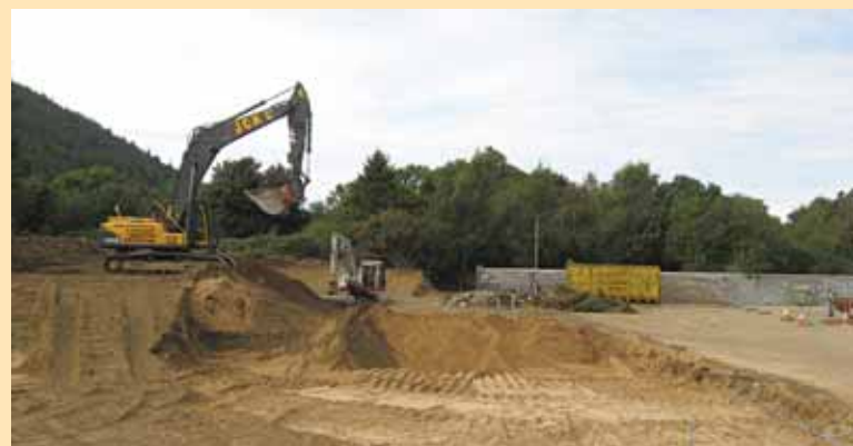
Sand was recycled as aggregate.
